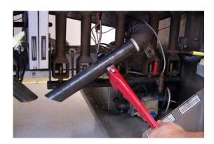
Removing 1.5" drain extension. (Step 19.A)
